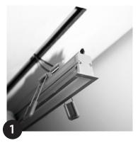
Cut 18 -22 mm (0.71-0.87") slot to required length. Bring through power feed and make connection to LINI-R.
